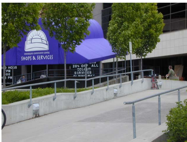
Accessible ramp at the University Community Centre Photo courtesy of Terri Tomchick-Condon
