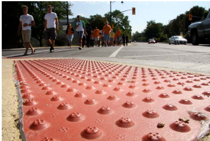
Photo of new detectable warning surface at road crossing. Courtesy of Paul Mayne, Western News
